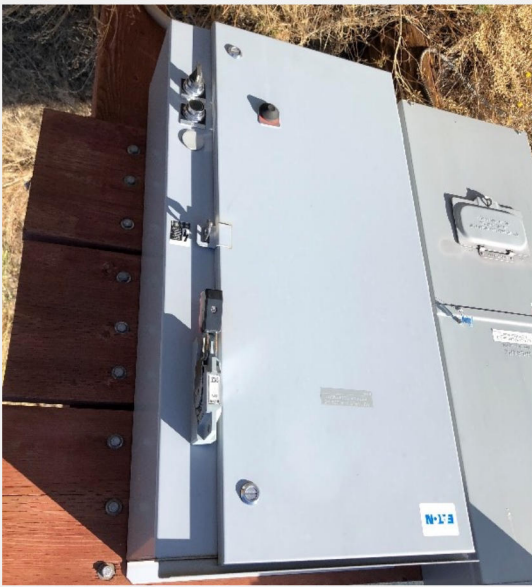
Photograph 2. Power and well control box adjacent to the onsite groundwater well.
