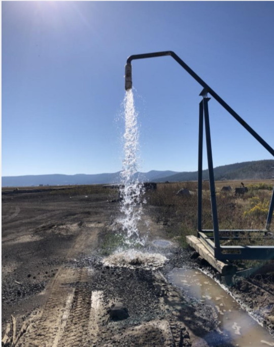
Photograph 5. Onsite groundwater well connected to J-stand for filling up water trucks. The onsite well was turned on during the site visit to confirm well operation and visually estimate flow rate.
