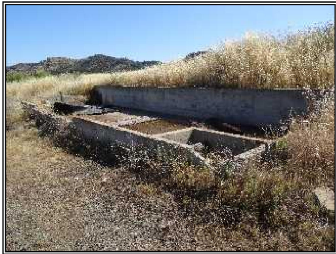
Looking a concrete feature to the northeast of the concrete pad.
