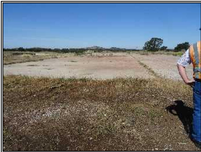
Looking at a concrete pad on the north-central portion of the Site.
