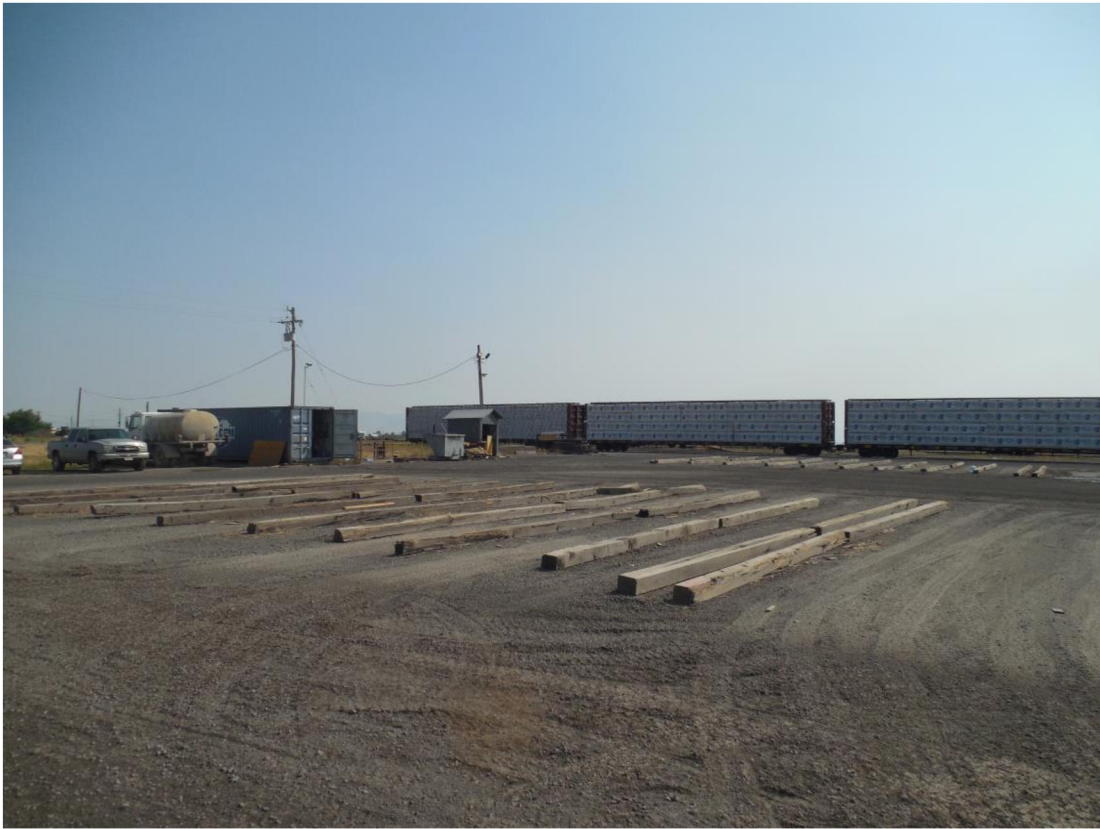
Rail loading area looking northeast
