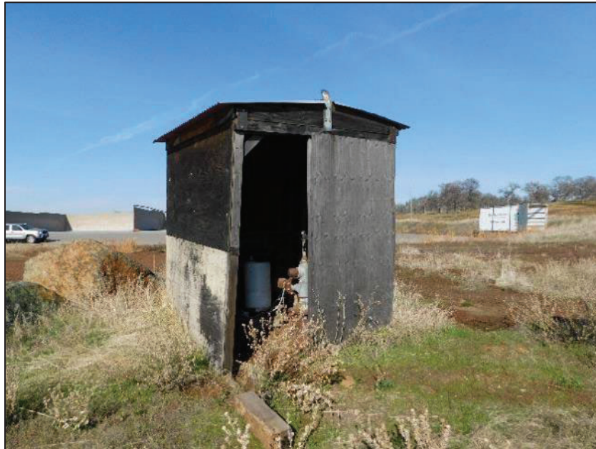
Exhibit 3. Component 3, Shed, view to northwest (Dudek image DSCN8042).
