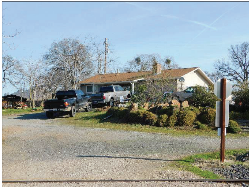
Exhibit 13. Component 13, Residence, northwest elevation, view to south (Dudek image DSCN8069).
