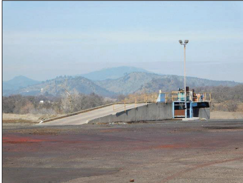
Exhibit 8. Component 8, Loading Dock, view to northwest (Dudek image DSCN7968).
