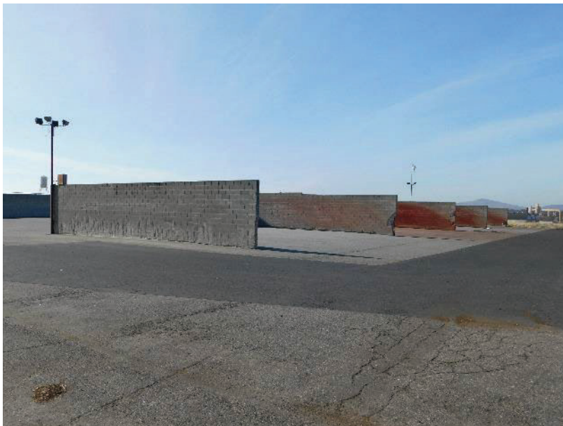
Exhibit 4. Component 4, Stalls, view to southeast (Dudek image DSCN7837).
