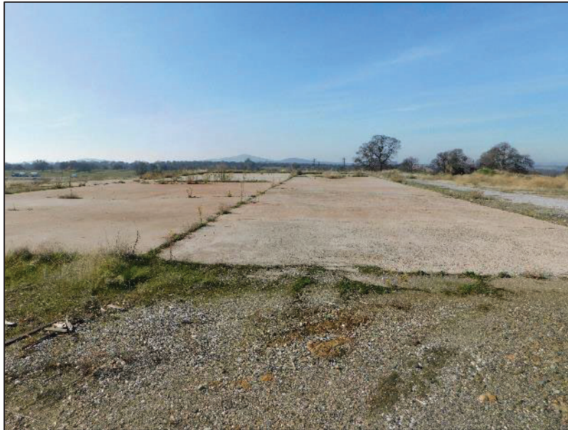
Exhibit 9. Component 9, Foundation, view to west (Dudek image DSCN8012).
