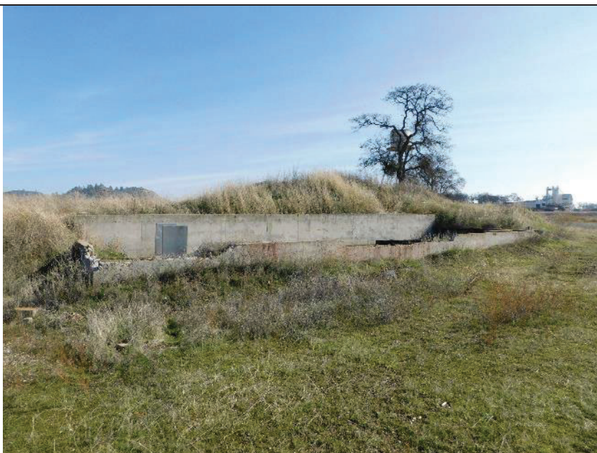
Exhibit 10. Component 10, Foundation, view to east (Dudek image DSCN8005).
