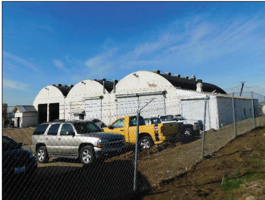
Exhibit 15. Component 15, Warehouse, south and east elevations, view to northwest (Dudek image DSCN8102).
