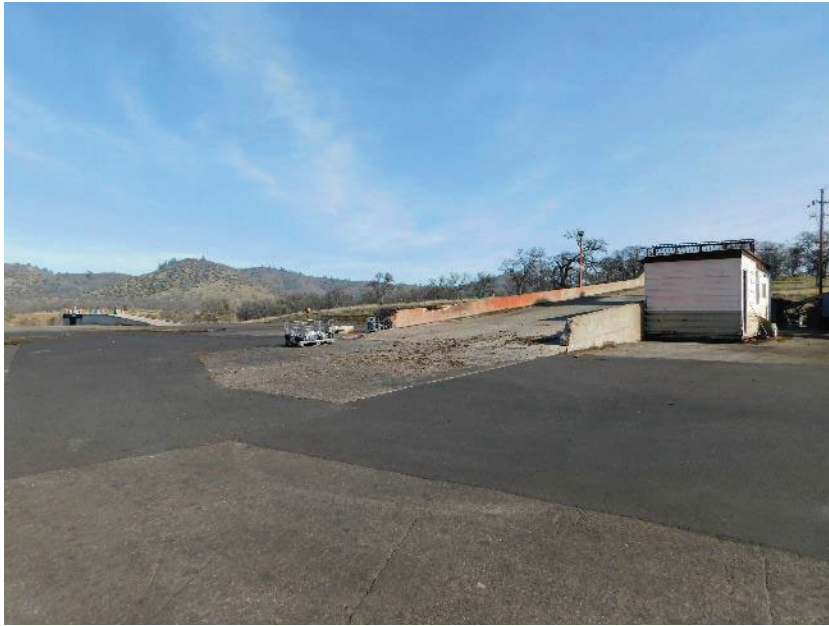
Exhibit 7. Component 7, Loading Dock, view to northeast (Dudek image DSCN7926).
