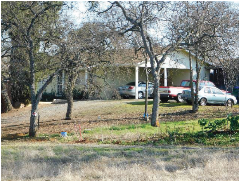
Exhibit 12. Component 12, Residence, north and west elevation, view to southeast (Dudek image DSCN8060).
