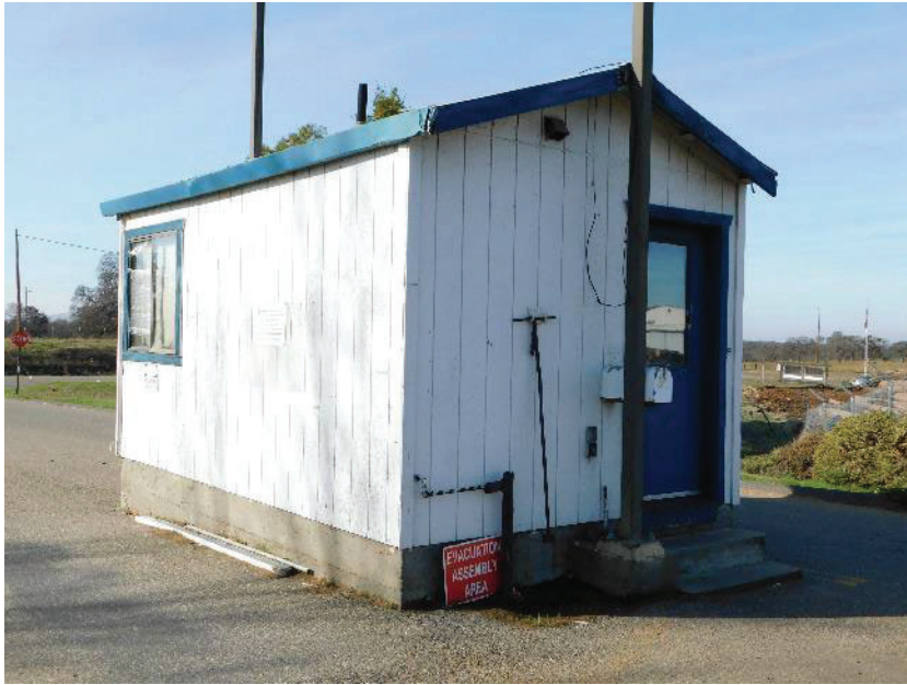
Exhibit 1. Component 1, Entrance Station, northeast elevation, view to southwest (Dudek image DSCN7793).
