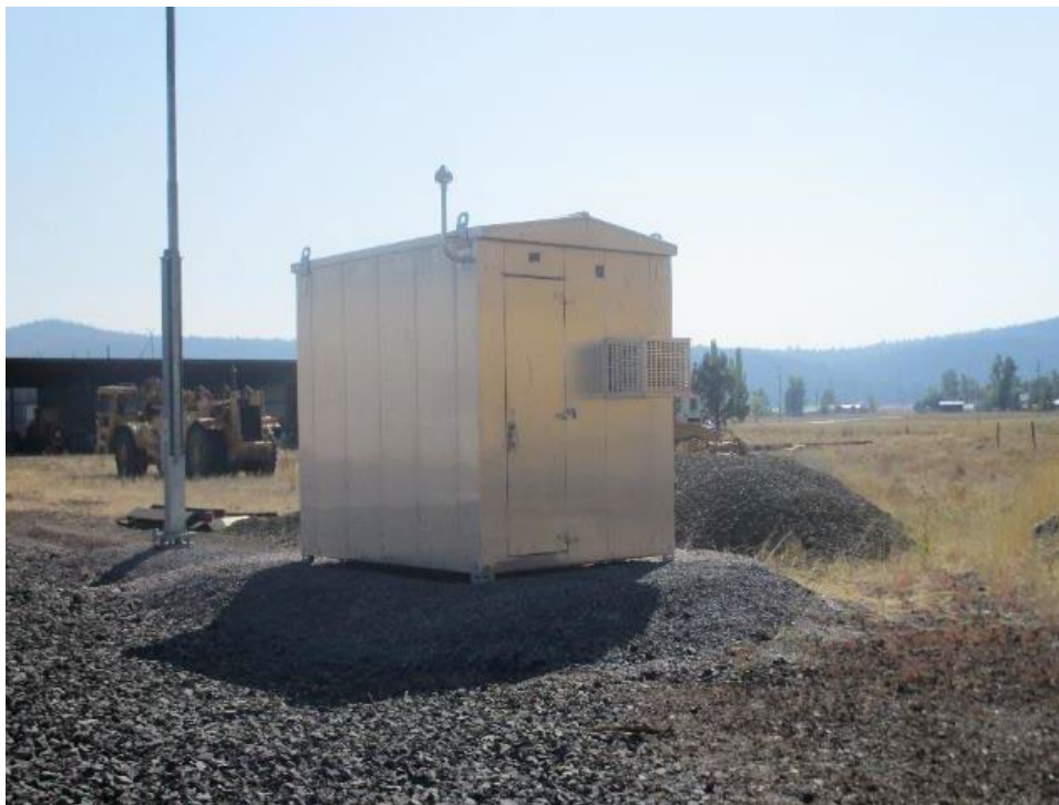
Photograph 28. The Electrical Shed, view looking southwest (IMG_521).
