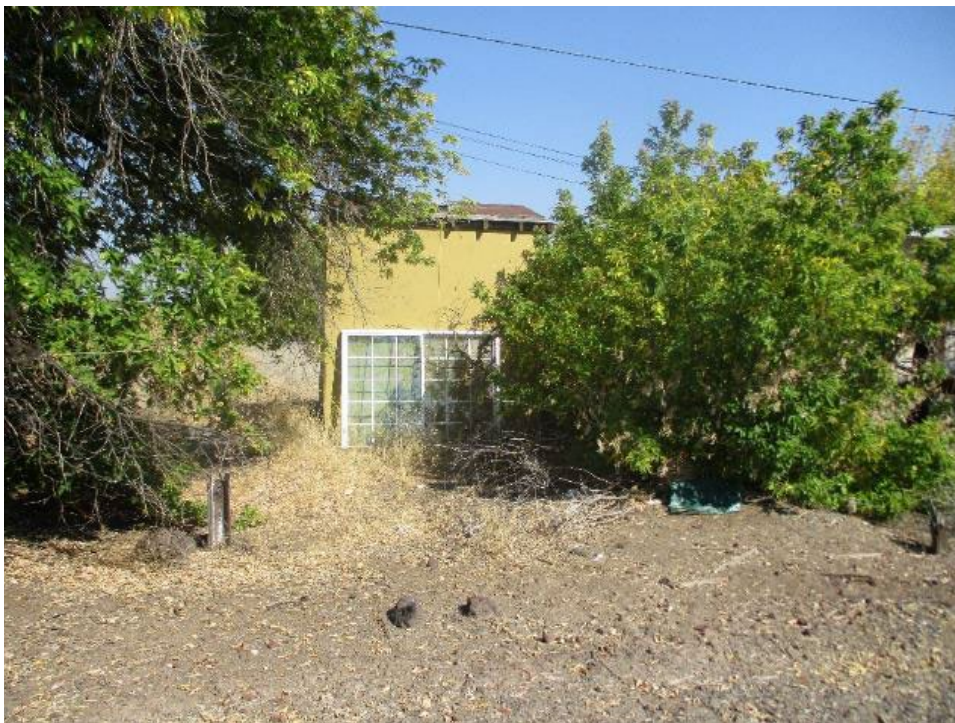
Photograph 29. The Shed, view looking east (IMG_531).
