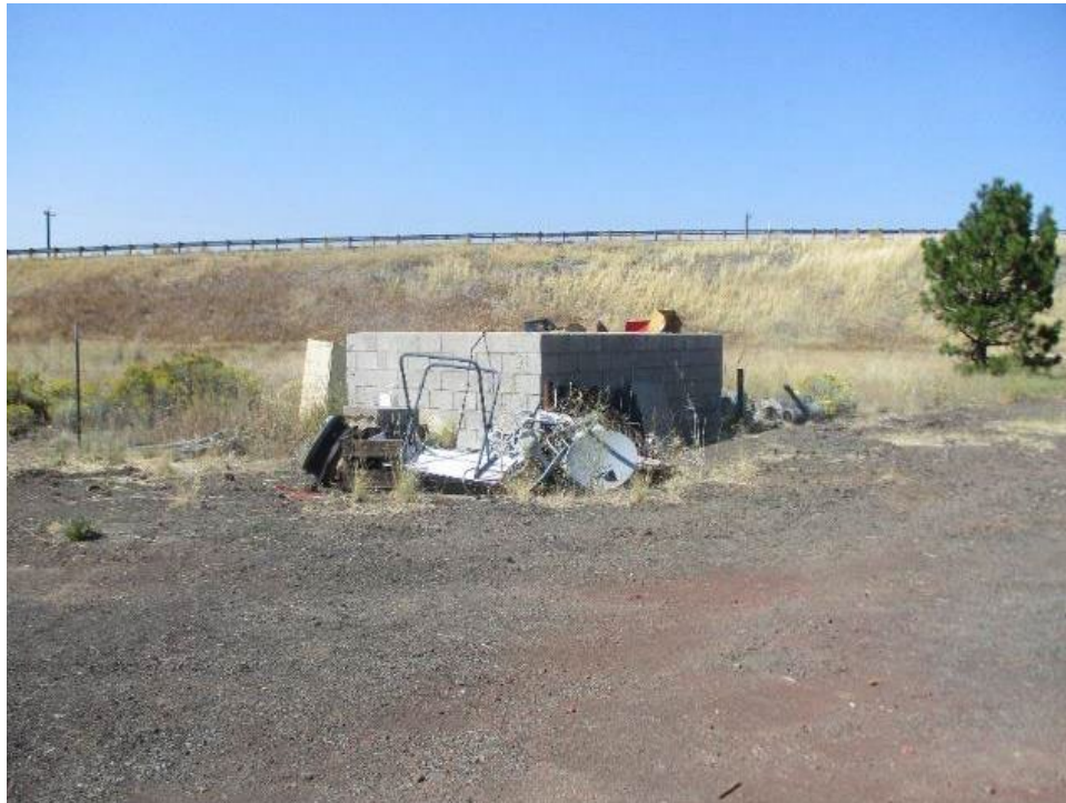
Exhibit 11. Map ID. 1E, Concrete Masonry Unit Structure, view looking north (IMG_472).
