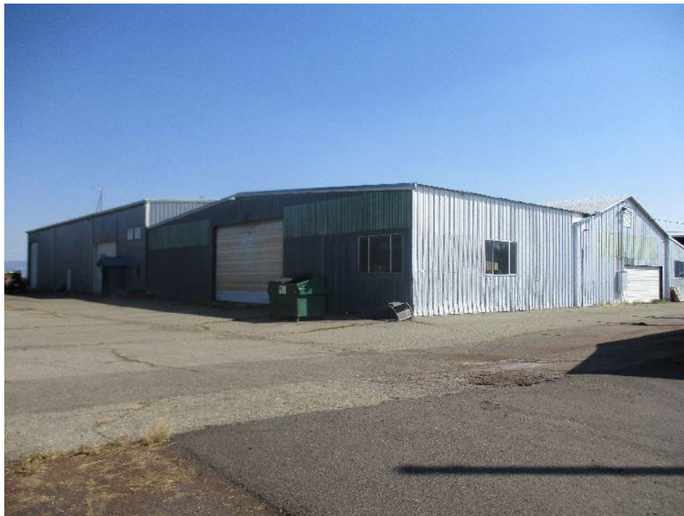
Exhibit 5. Map ID. 1C, Warehouse, north and west elevations, showing multiple additions. View looking southeast (IMG_483).
