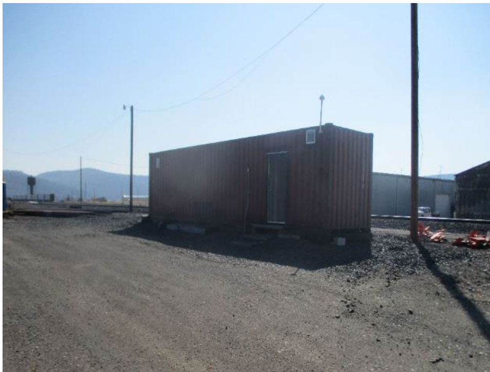
Photograph 25. Shipping Container Storage Building, view looking southwest (IMG_529).
