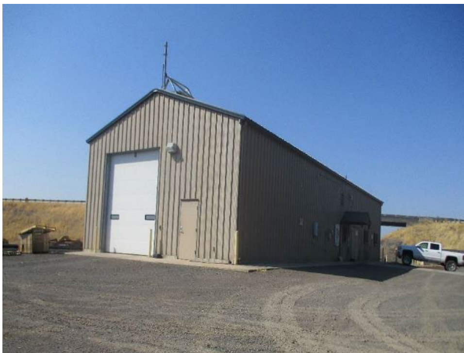
Photograph 23. The BNSF Railroad Administrative Office, view looking northwest (IMG_515).
