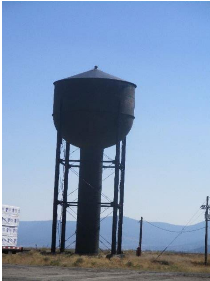
Exhibit 16. Map ID. 2B, Water Tower, view looking southeast (IMG 445).
