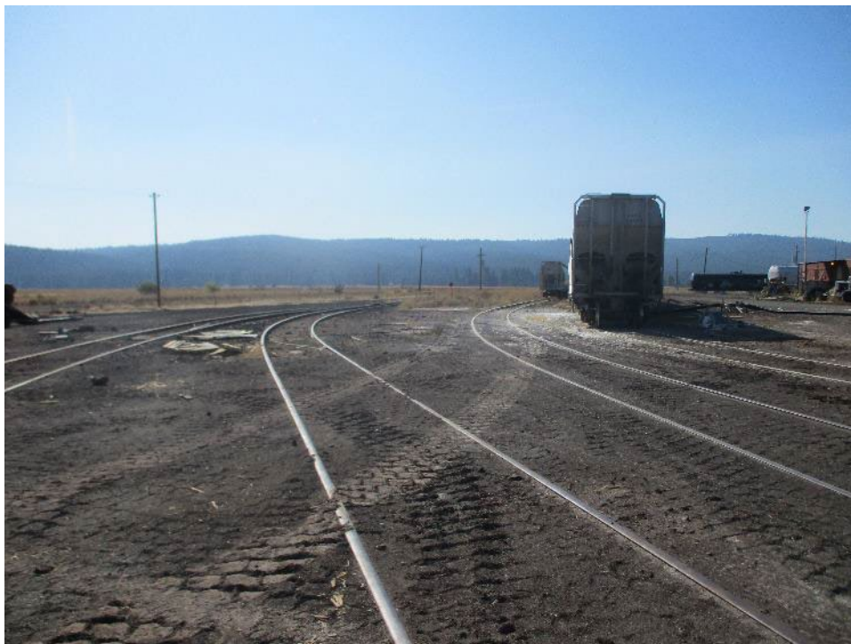
Photograph 15. Railroad spur lines, view looking west (IMG 555).
