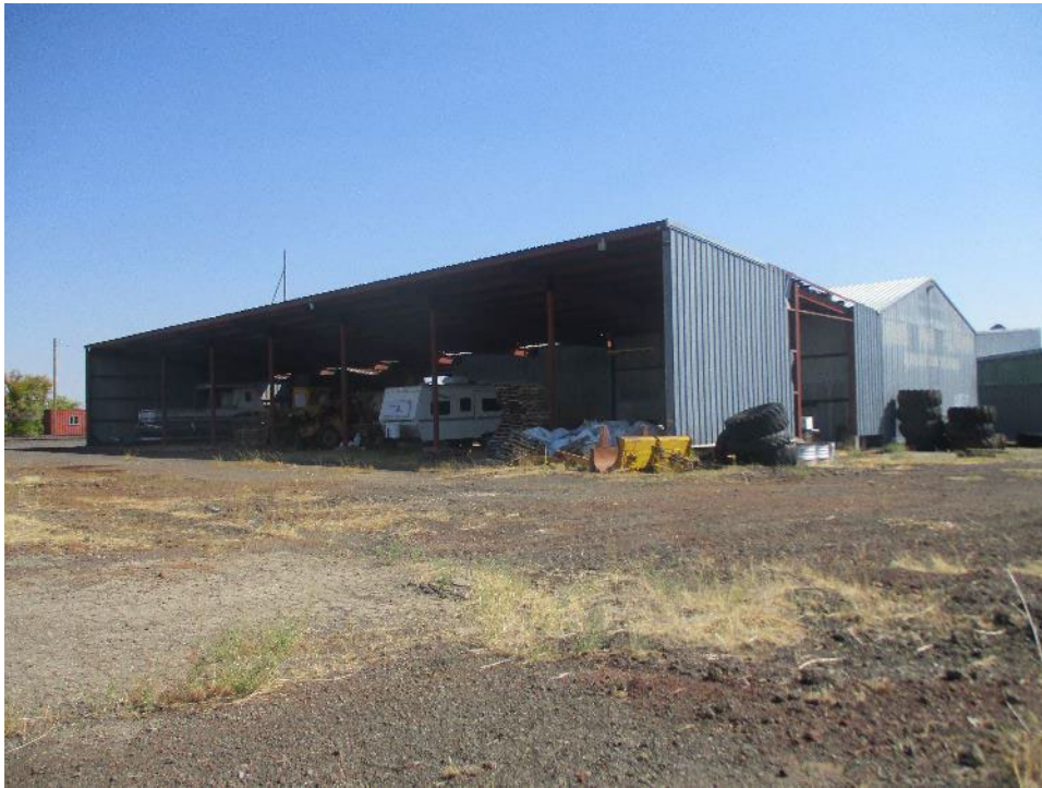
Photograph 3. Storage Barn A, view looking southeast (IMG_474).
