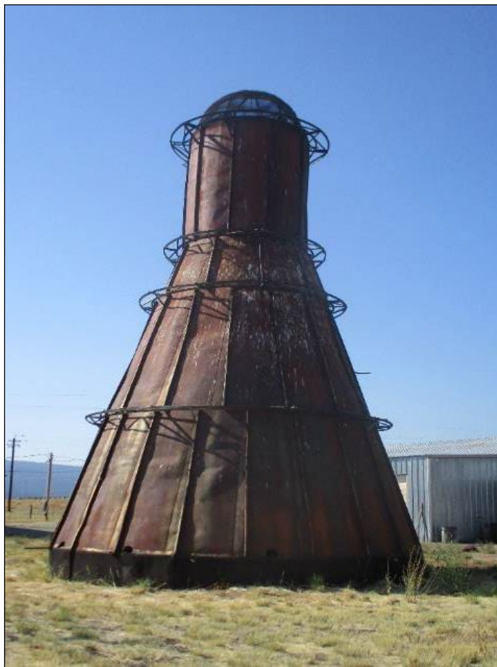
Photograph 9. The Silo, view looking west (IMG_511).
