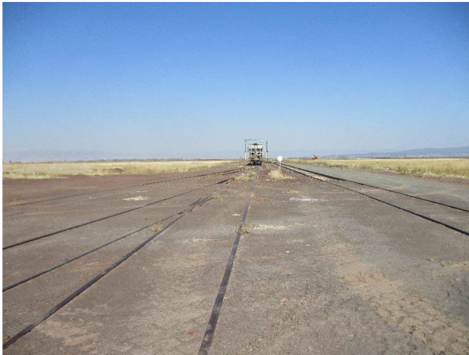
Photograph 14. Railroad spur lines, view looking east (IMG 554).
