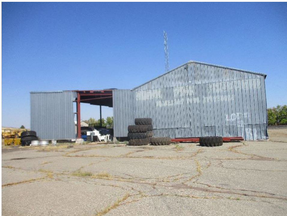
Photograph 4. Storage Barn B, view looking east (IMG_481).
