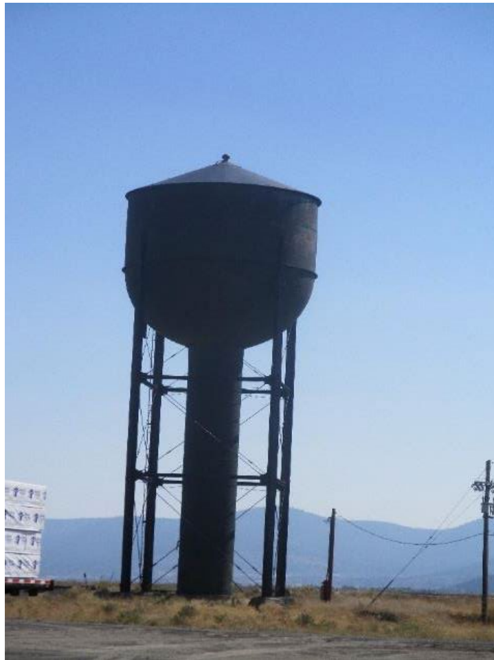
Photograph 16. The Water Tower, view looking southeast (IMG 445).
