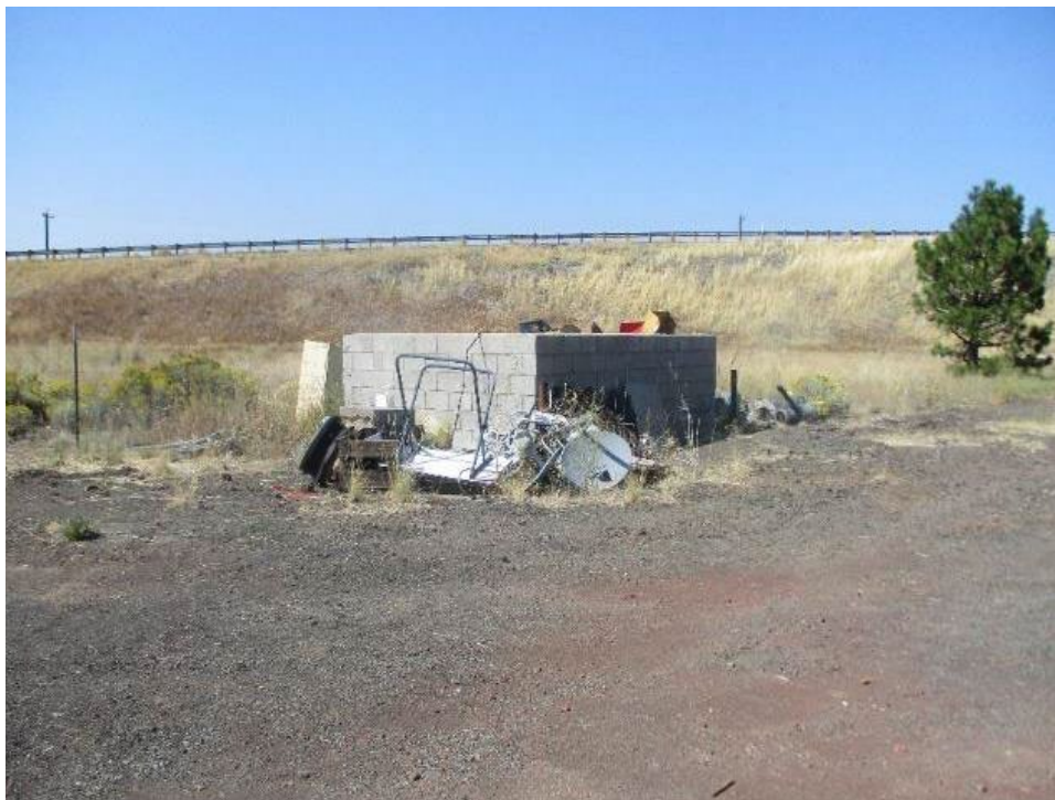
Photograph 11. The Concrete Masonry Unit Structure, view looking north (IMG_472).
