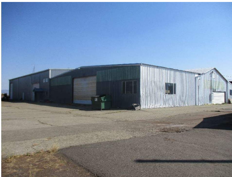
Photograph 5. The north and west elevations of the Warehouse. View looking southeast (IMG_483).
