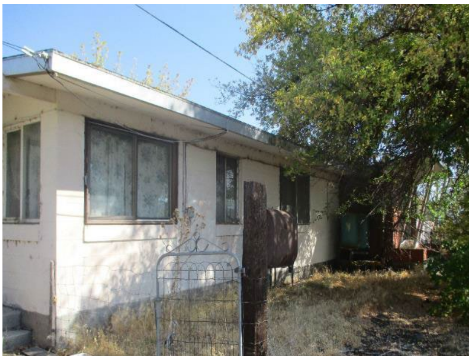
Photograph 18. The GNWP Railroad Depot, view looking southeast (IMG_534).
