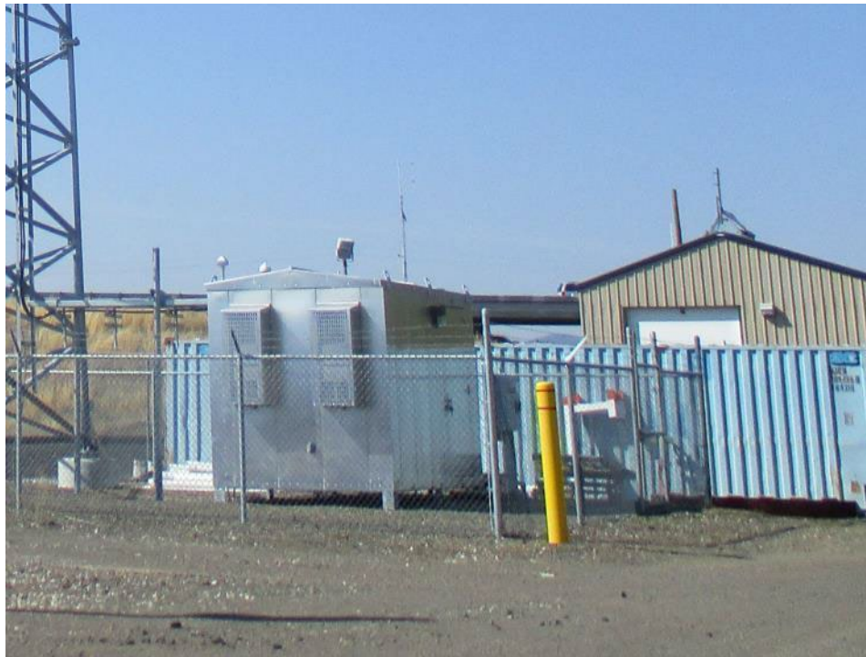
Exhibit 27. Map ID. 2I, Shipping Container Storage Building (right), view looking north (IMG_526).
